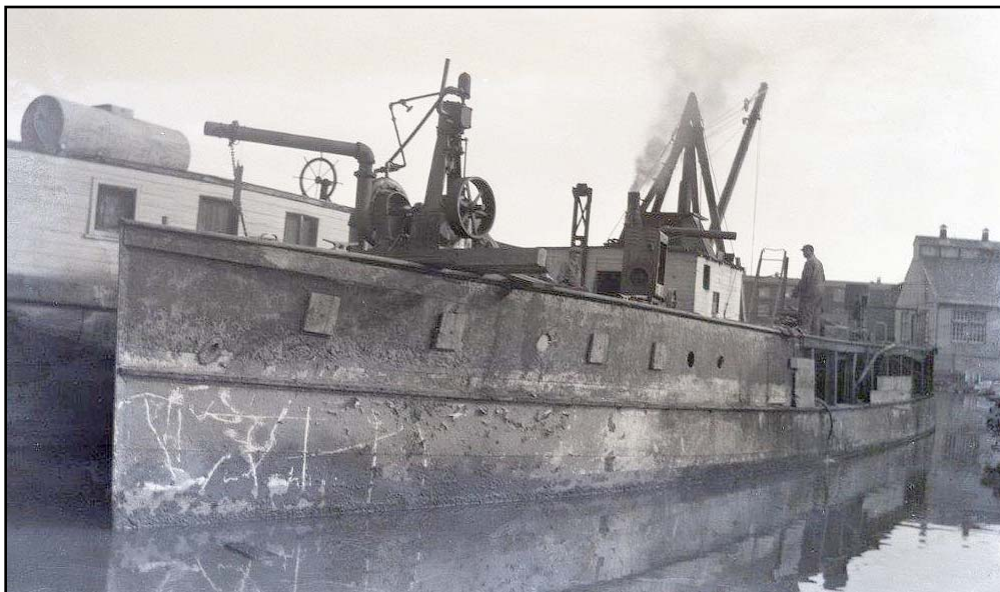
Front View, floating beside “Filgate” with the steam pump still on deck.
