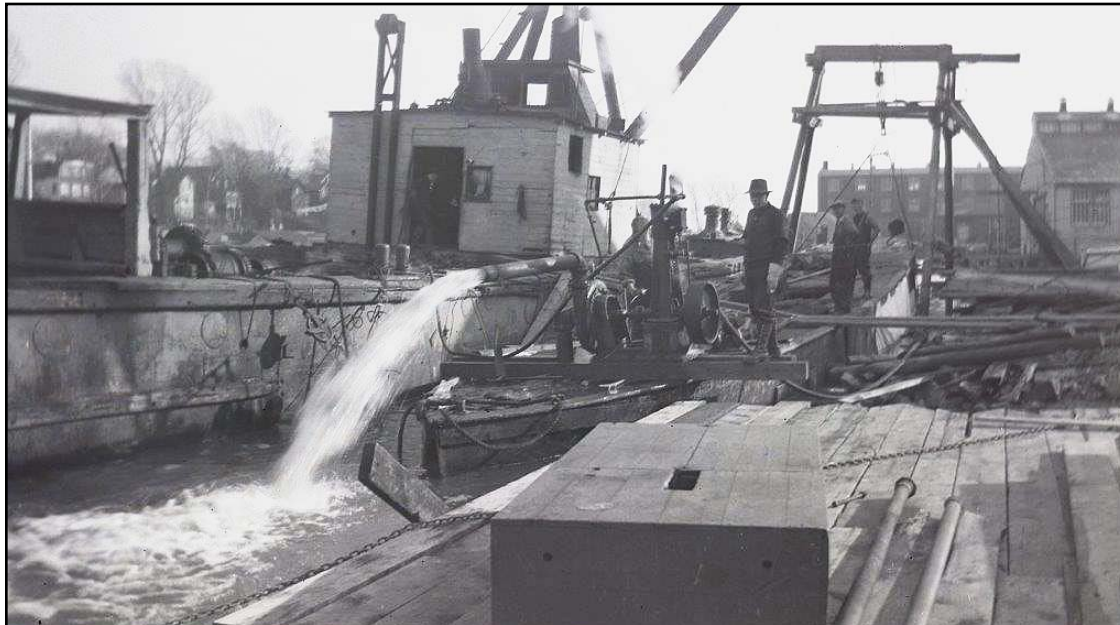
The stern is hoisted on a gantry, while a stream pump is used to lighten the bow. About 26 November, 1948
